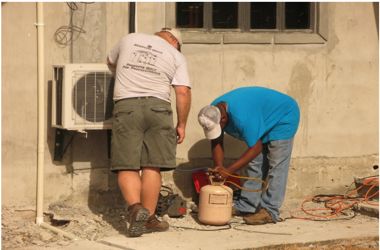
Time to charge new cooling split system
