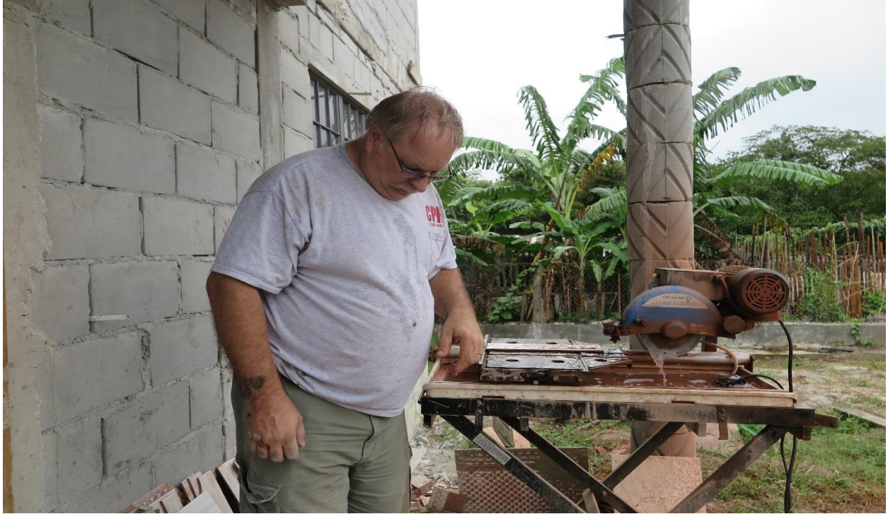
Jonathan getting ready to cut some tile.
